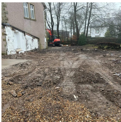
Cleared footprint following demolition
