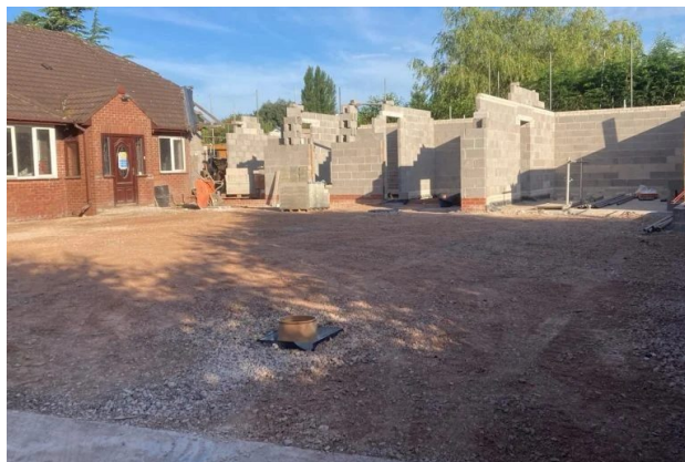
Blockwork during construction
